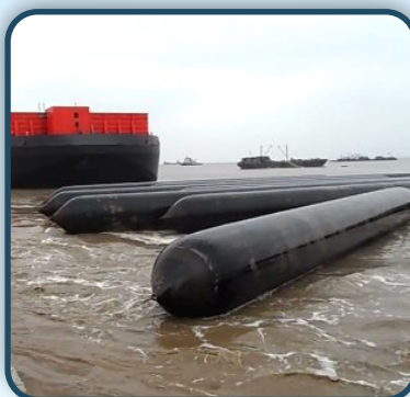
Ship Launching Airbags
